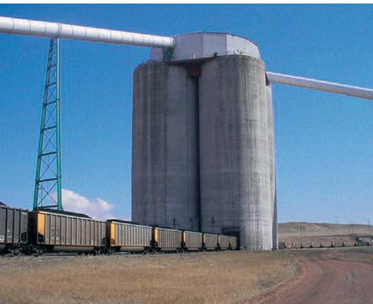
High capacity western U.S. surface mines, such as Cordero Rojo's loading system pictured above, have played an integral role in the evolution of unit train loading systems.
